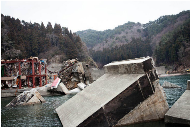
Figure 47: The Kamaishi breakwater, which failed during the 2011 Japanese tsunami (NY Times)
