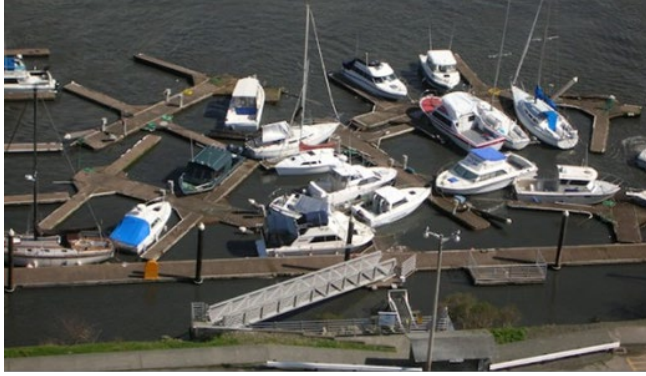
Figure 10: Docks broken from Japan 2011 distant tsunami in Brookings OR. (USCG / Group Air Station North Bend)
