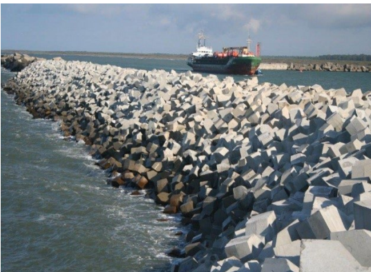
Figure 49: Photo of fortified breakwater off marina.
