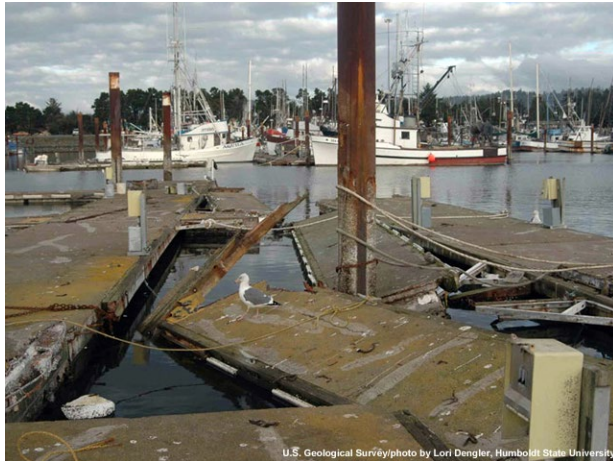
Figure 45: Broken docks in Crescent City, CA from the 2006 Kuril earthquake (USGS 2006).
