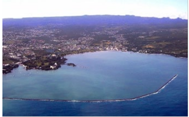
Figure 50: Breakwater protecting the harbor of Hilo, Hawaii (Big Island Gazette)
